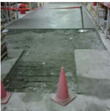
Floor Restoration System
