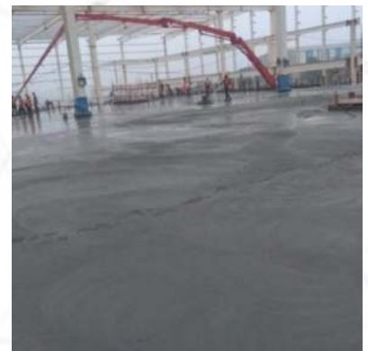
Post Tensioned Jointless slabs
