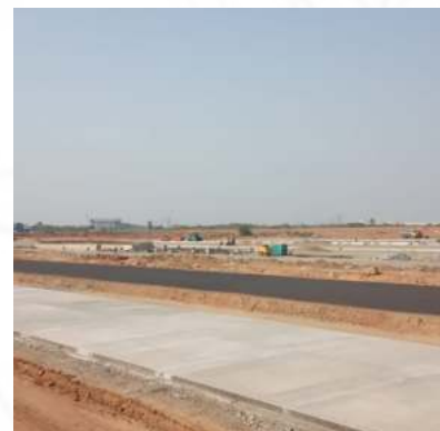
PQC Roads & Pavements
